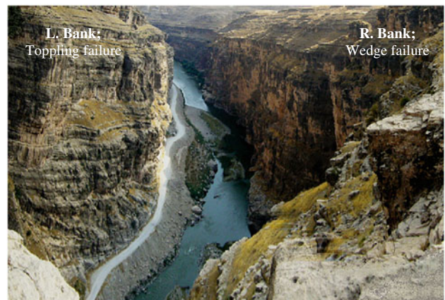
Fig. 17 U shaped valley downstream of Seymareh River with near vertical cliffs. Kinematic analysis indicates rock instabilities at right and left flank are mainly wedge and toppling, respectively
