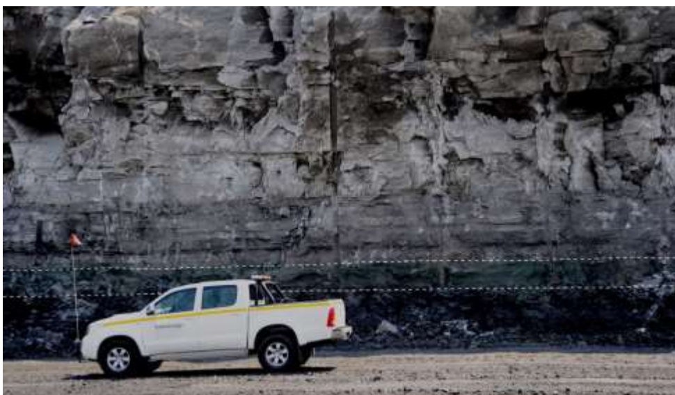
Fig. 15. Thick (0.90 m) development of the Glauconitic Sandstone Marker (between the dotted lines) above the No. 5 Seam in the Delmas region of the Witbank Coalfield. Keaton Energy's Vanggatfontein Colliery.
