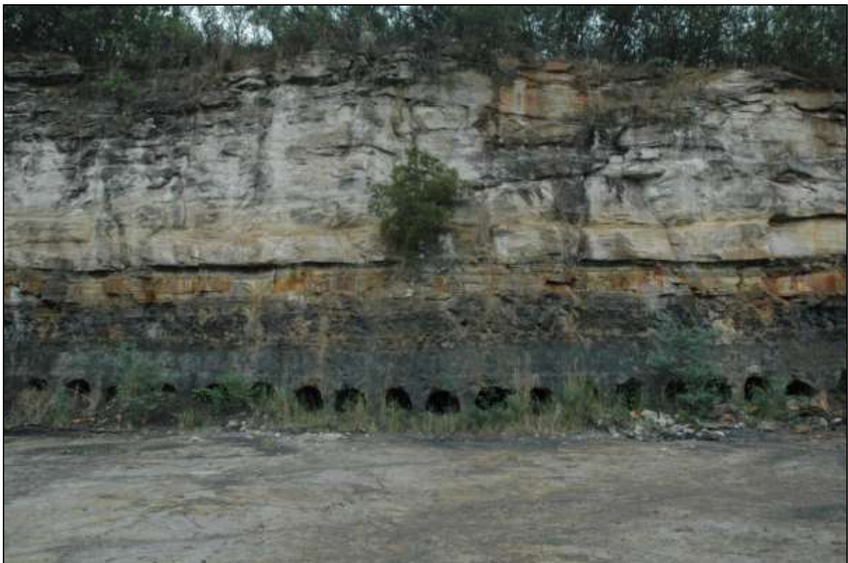
Fig. 29. Local stratigraphic succession in the historic contour surface mine (Pit A; old D and G workings) on the farm Vryheid 159, showing the holes in the lower part of the Alfred Seam left by the auguring operations.
