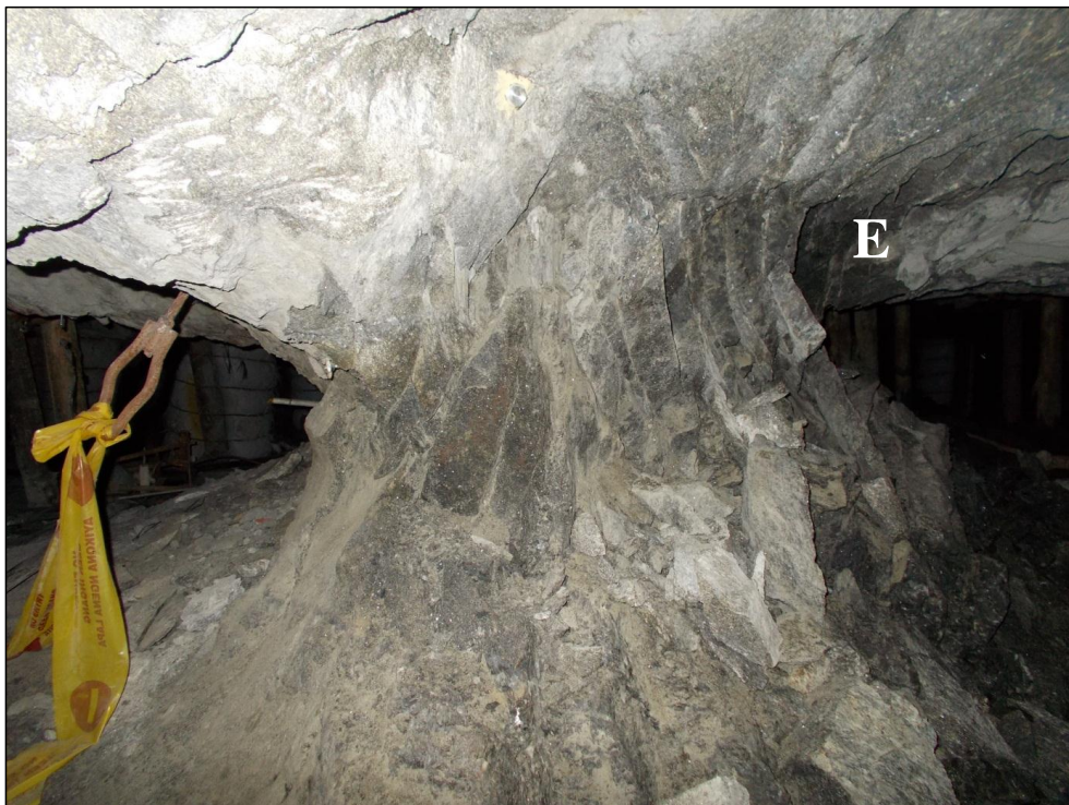
Figure 8.29: Down-dip view of pillar P1. Notice the intensity and spacing of the fractures towards the eastern side. Photograph taken on 23 April.
