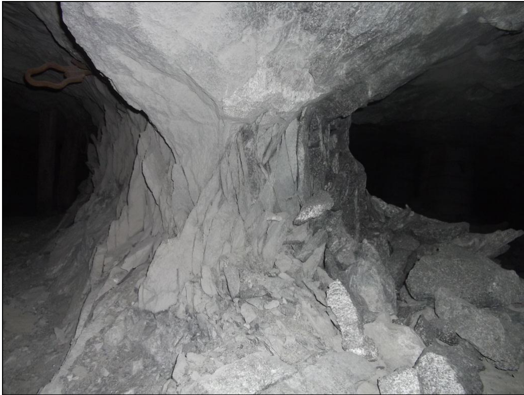
Figure 8.16a: Pillars consisting of mostly Anorthosite hangingwall (pillar 6). Note the difference in fracture intensity compared to Figure 8.16b below.
