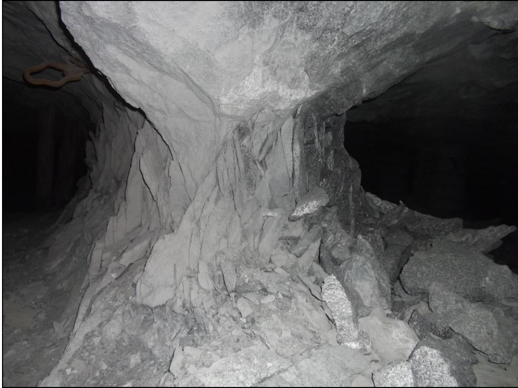
Figure 8.46: Wedge like formation along the down dip side of pillar 4 where the fractures intersect.
