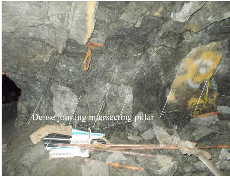
Figure 8.35: Dense jointing intersecting pillar P3. Photograph of the bottom down-dip portion along the western side of the pillar.
