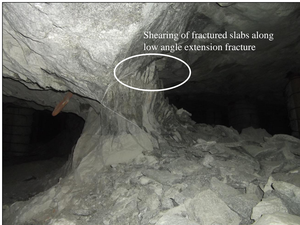
Figure 8.49: Shearing of fractured slabs along low angled extension fracture (down-dip side of pillar 5).
