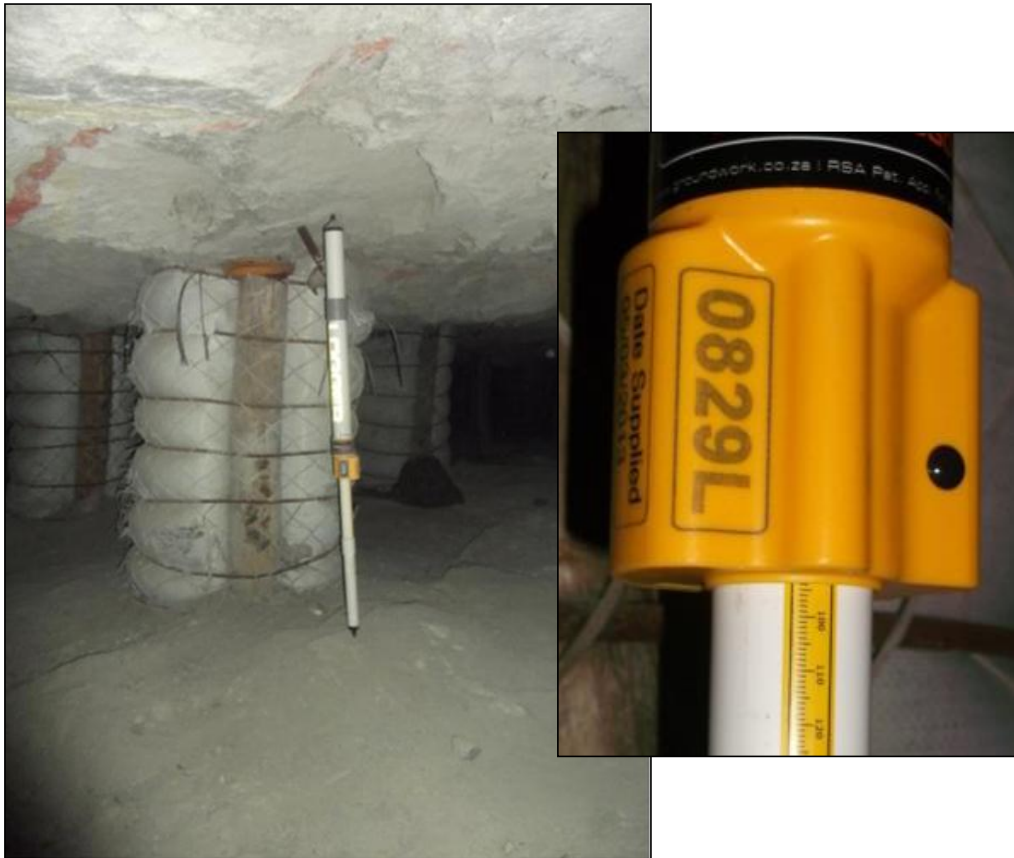
Figure 9.7: A closure logger measuring continuous convergence in the trial site.
