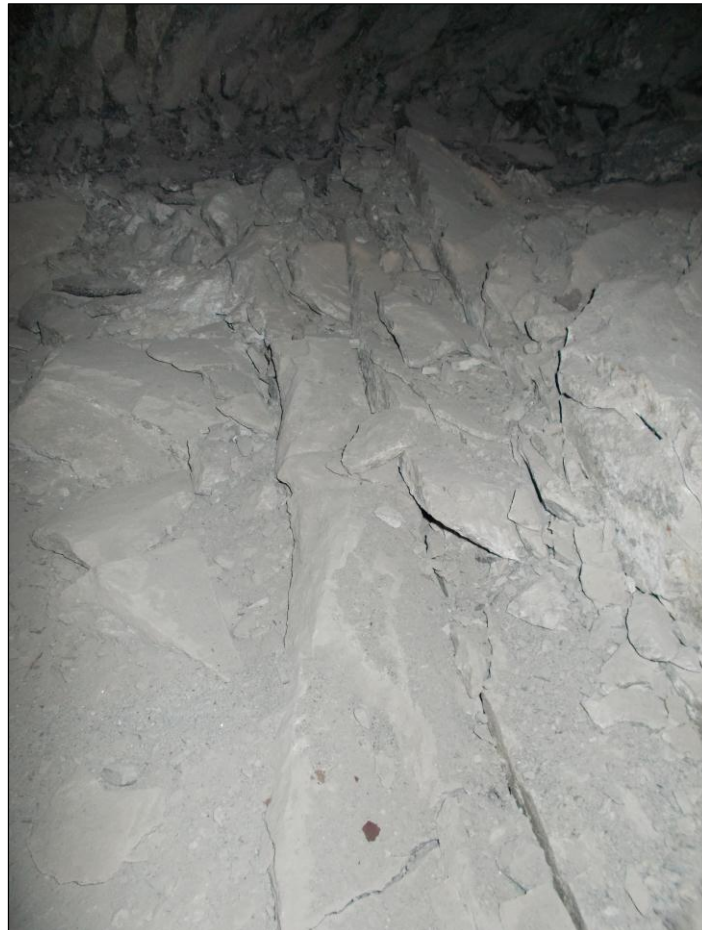
Figure 8.20: Footwall heave experienced adjacent to the west side of pillar 42.
