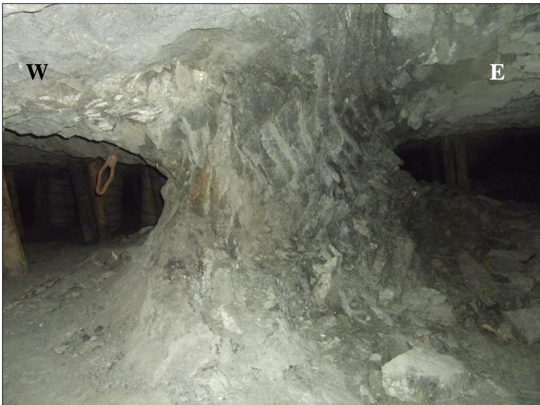
Figure 8.12b: Pillar scaling towards the east. Photograph of the up-dip side of pillar P1.
