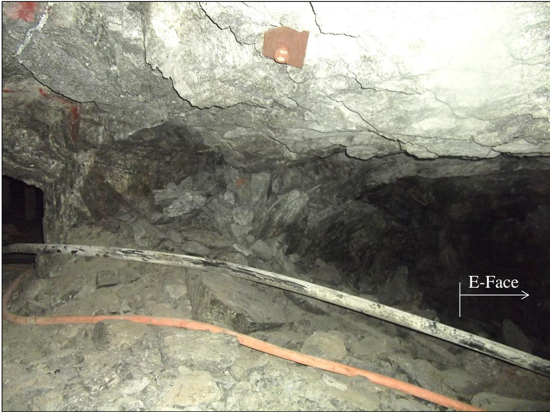
Figure 8.19: Condition of pillar 37 whilst still part of the mining face.
