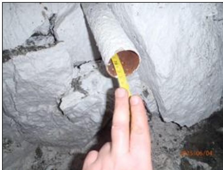
Figure 9.35: Photograph of tape extensometer installed in horizontal borehole through pillar P2.
