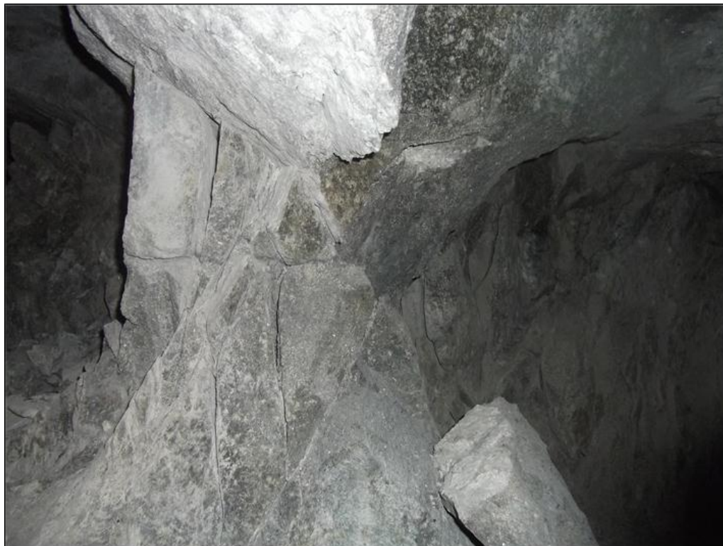
Figure 8.47: Wedge like formation in the centre of a pillar (pillar 43 up-dip view).
