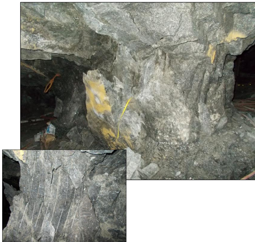
Figure 8.34: Down dip view of the top and western side of pillar P3. Bottom insert indicates the degree of fracturing along the top western side of the pillar (see white line traces along the bottom of the pillar). The photograph was taken on 6 May.
