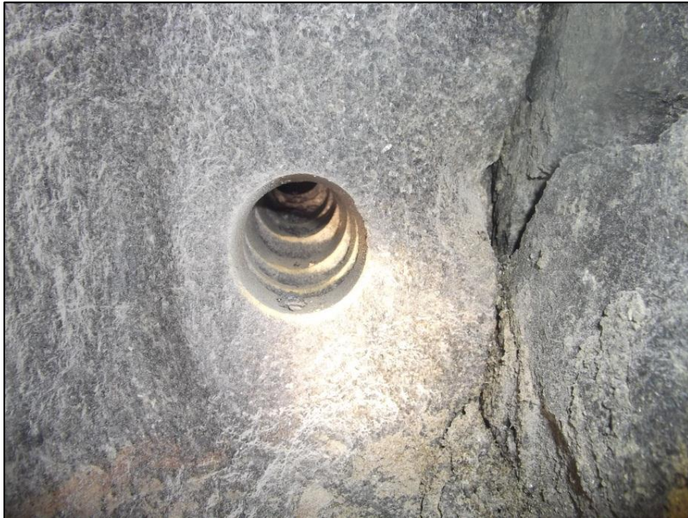
Figure 8.31: Photograph of a borehole through pillar P2. Note how the slabs defined by the fracture planes have moved relative to one another. The photograph was taken on 16 March prior to the formation of the pillar.
