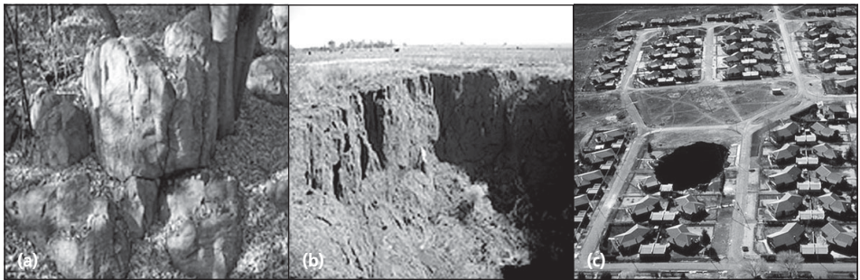
Figure 7 Sinkholes that developed near Carletonville.
