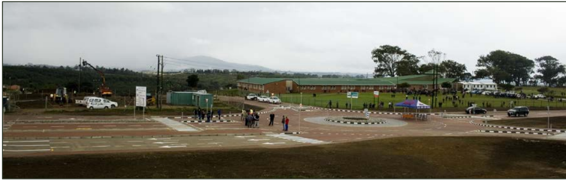
Figure 3: Traffic circle to accommodate bus turning & terminus facilities – Thembaletu (Source: George Municipality CES)
