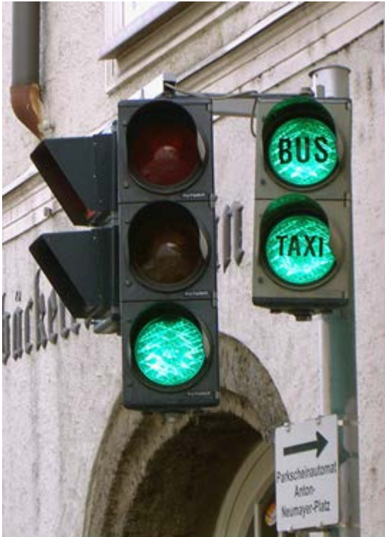
Figures 2a and 2b: Examples of BRT signals with bus profiles in the lenses found in Salzburg, Austria and Swansea, Wales respectively (Ref 2)
