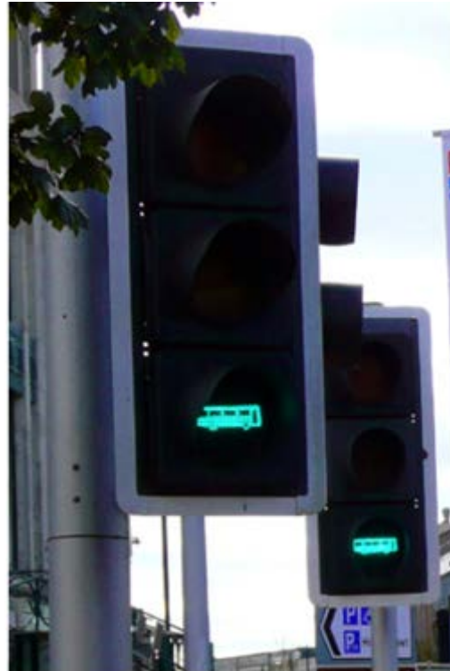
Figures 2a and 2b: Examples of BRT signals with bus profiles in the lenses found in Salzburg, Austria and Swansea, Wales respectively (Ref 2)
