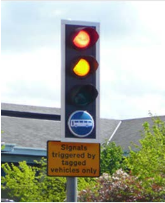
Figures 4a and 4b: Examples of BRT signals similar to normal signals with supplementary signs found in North Kent, England and Schaffhausen, Switzerland (Ref 2)
