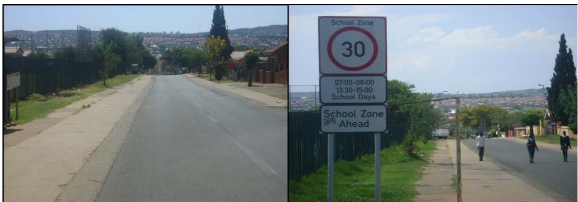
Photo 1: Before - Maboea Street Direction North
