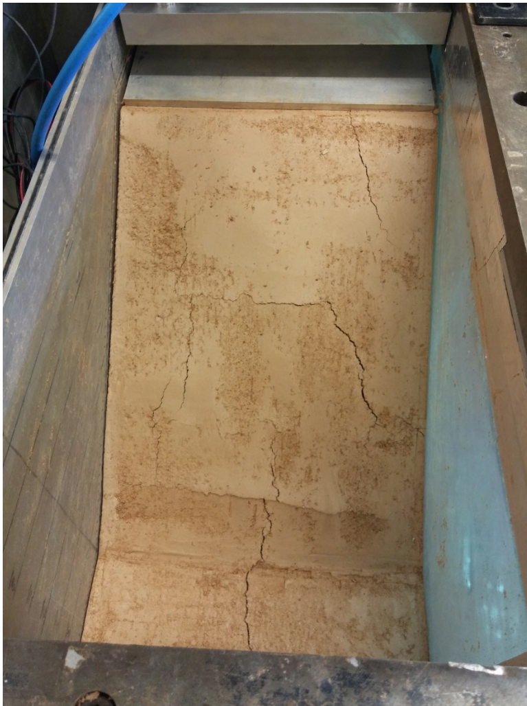
Figure 4.30: Cracks that formed on the face of the embankment with Test B6 (23.0 % MC)
