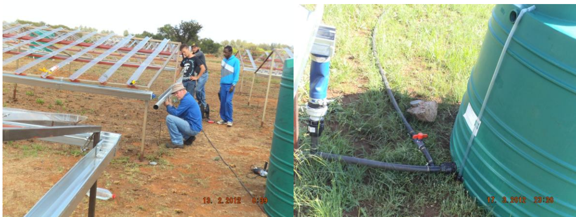
Figure 5.1 Rainout shelter structure (rainout shelter, left; Jojo tanks for water collection, right) at Hatfield Experimental farm, Univeristy of Pretoria
