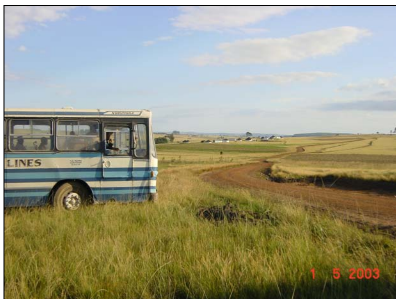
Figure 2. The finished road - a bus service has been introduced.
