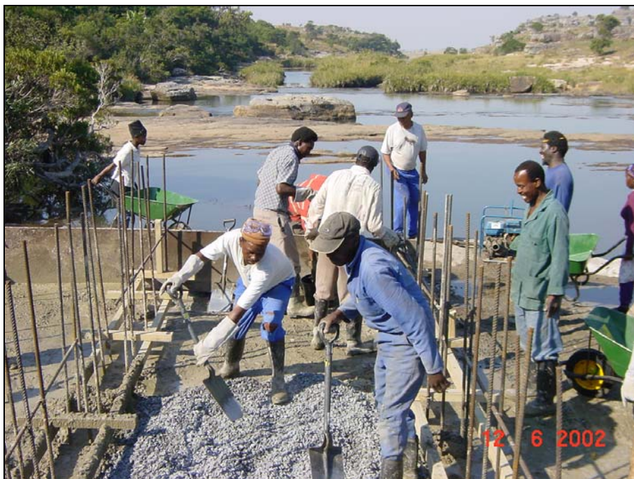
Figure 5. Training in concrete batching and placing.
