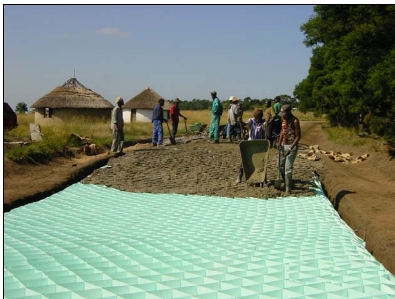
Figure 4. Concrete geocell drift under construction.
