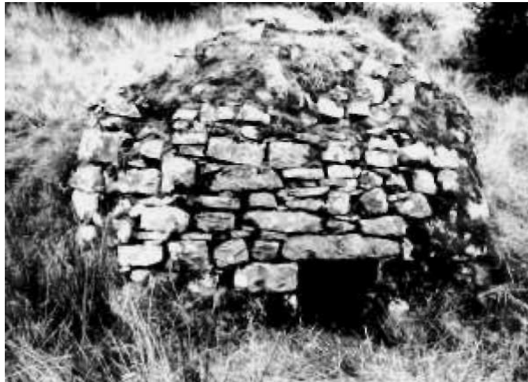
Figure 8 A corbelled Irish sweathouse (Weir, 2007).
