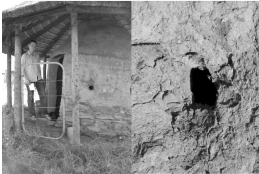
Figure 9 & 10 Voorhuis charcoal burner, entrance and close up of tuyere aperture (Fisher 2007).
