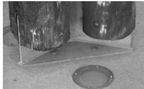
Figure 6b Coexistence of different materials and technologies, columns, Red Location, PE.
