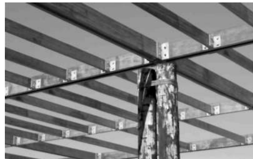
Figure 6d Gum poles and industrial timber, steel and ropes, Red Location Museum, PE.
