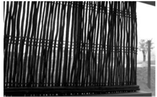
Figure 8b Details of screens made of available materials, hotel in Maropeng.
