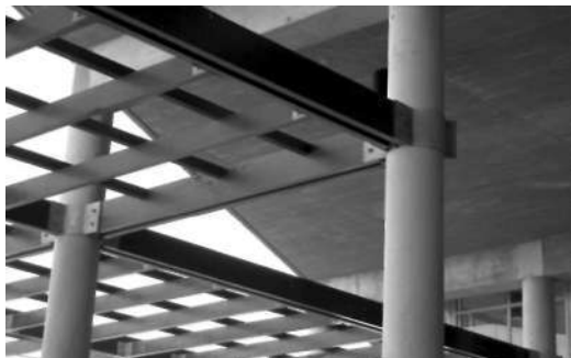
Figure 6c Concrete columns, steel joints and industrial timber, Red Location Museum, PE.
