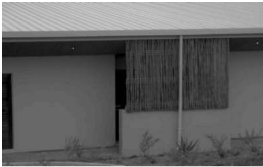
Figure 8a Screens made using available materials, skills and labour, hotel in Maropeng.
