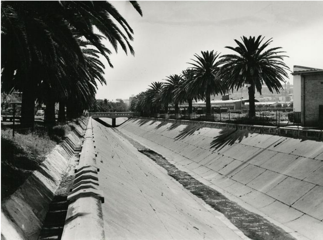
Figure 55: Canalisation of Apies River with bridge (1951) (Source: Anon, 2013o)
