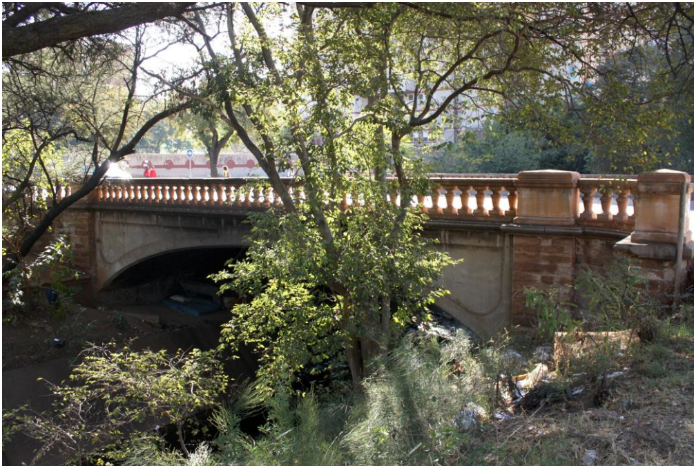
Figure 35: Victoria Bridge built in concrete as it is today (Source: ABLEWiki, 2009)
