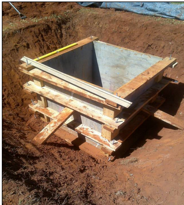
Figure 3.19: Excavated pit with formwork
