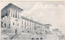
Pennsylvania State Capitol Building.
