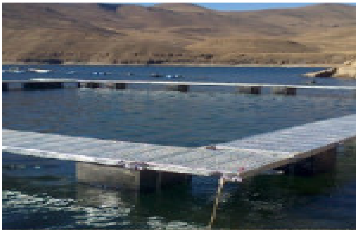
Figure 1.3: The rainbow trout farming cages in the Katse Dam (taken from Eilertsen, 2013)
