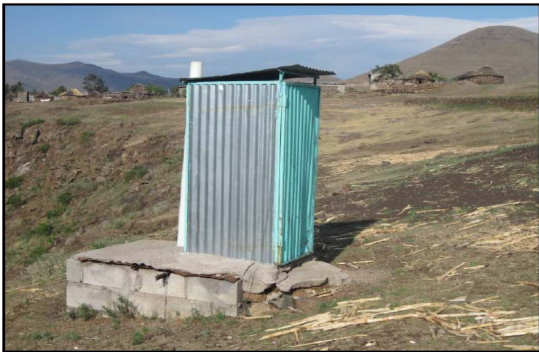
Figure 3.7: A pit-latrine used in the Thaba-Tseka District (adapted from Letsebe, 2012)
