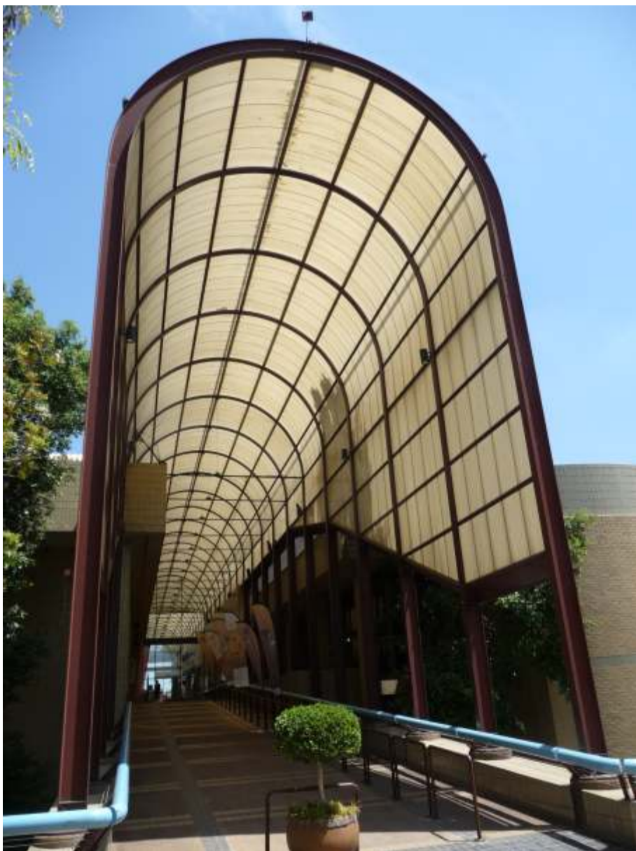
Figure 1.1.1. Ramped walkway to main entrance of the Ditsong: National Museum of Cultural History.
