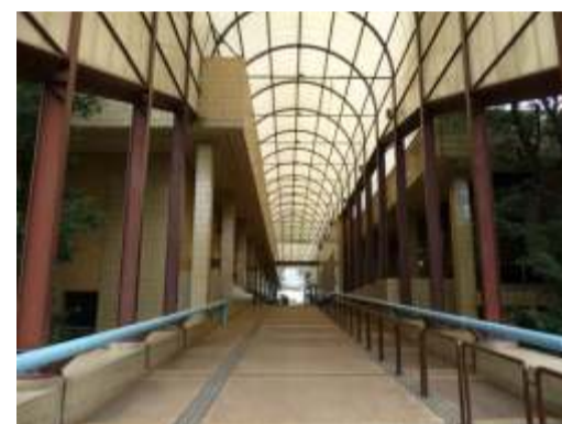
Figure 2.5.3.2. Ramped walkway to entrance.
