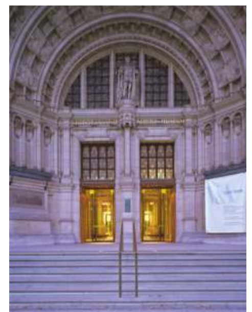
Figure 4.1.1.4. Cromwell Road entrance. (EJAL 2003).
