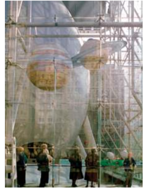
Figure 4.1.3.5. Balustrade with information panels visible at bottom of figure. (Ennead 2014).
