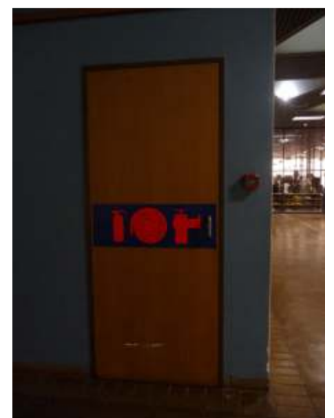
Figure 3.5.4. Evacuation route signage
