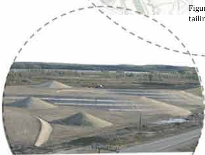
Figure_5.18. Mine reclamation at Mcleods tailings(MSP,2001)
