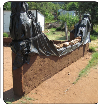
MUD PLASTERED ROCK WALL
