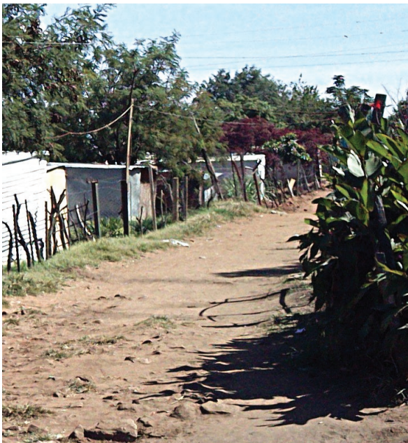
Figure 25 Much less erosion from roads running perpendicular to the mountain's slope (Author 2015)
