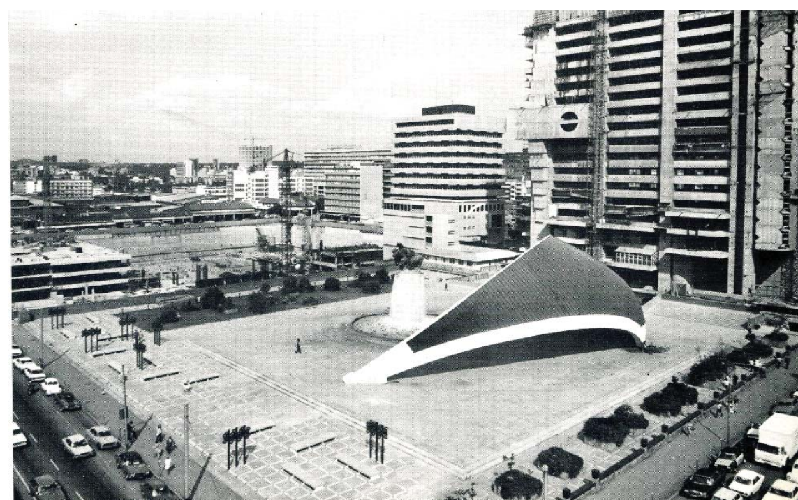
Figure 2.6 - State Theatre and Volkskas Bank in construction.psd
