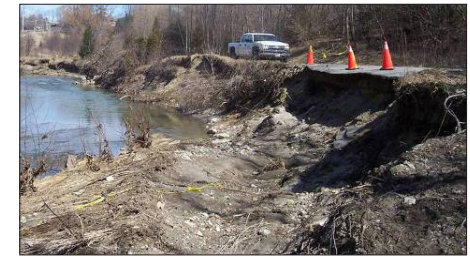
Photo 1.3.10: Prior to rehabilitation
