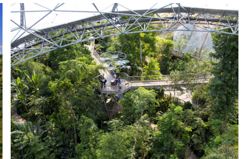
Fig 2.24: Eden project biomes (The Eden Project 2001)
