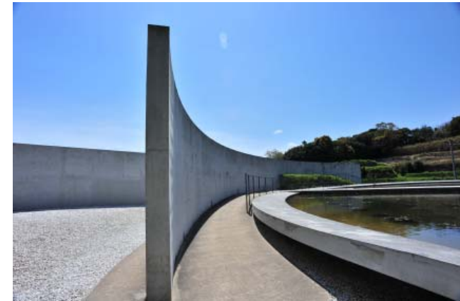
fig 9.6. Concrete wall that exposed views of Pond and site that on plan related to the geometry of the entire project
