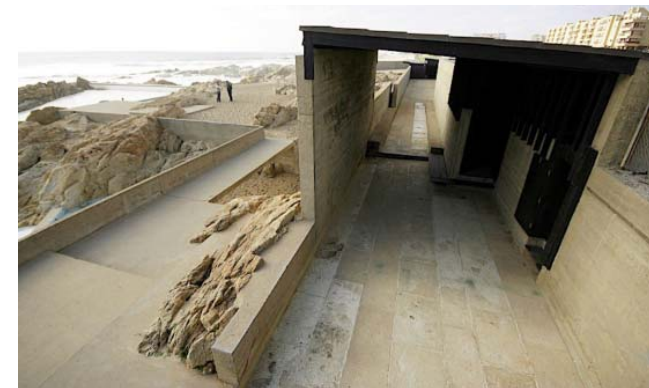
fig 9.15. Images depicting various thresholds throughout journey towards the ocean. As well as relationship between natural rock and concrete cast into one another.
