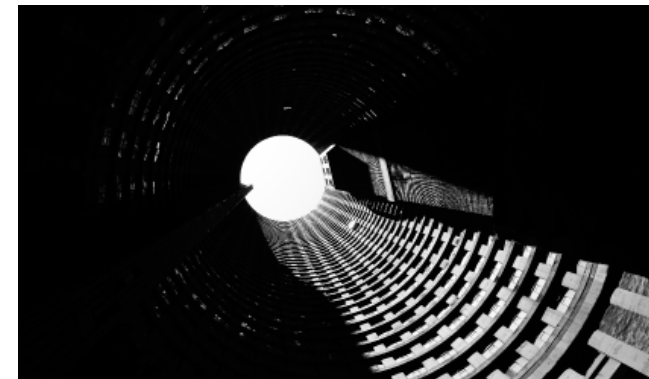
fig 5.5. Photographs of Ponte City taken during a tour of the structure explaining its history from during Apartheid until now. (by Author, 2013)
