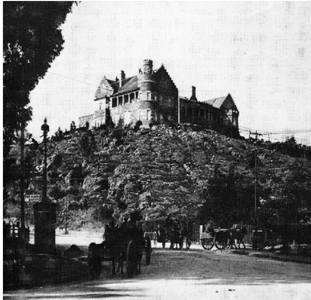
fig 3.6. Image of Eastington Manor from Saratoga Avenue.
