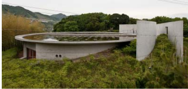
fig 9.8. Image showing relationship between concrete wall oval pond and staircase descending into it. It also shows the structures geometric relationship with the natural environment.
