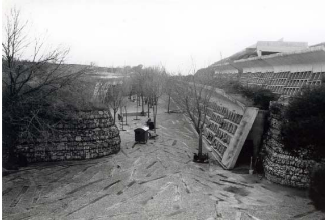
fig 9.4. Entrance into Iqualada Cemetery between Gabion walls that house the Graves and Circulation
