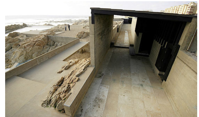
fig 9.15. Images depicting various thresholds throughout journey towards the ocean. As well as relationship between natural rock and concrete cast into one another.
