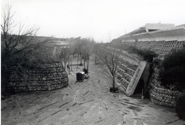
fig 9.4. Entrance into Igalada Cemetery between Gabion walls that house the Graves and Circulation
