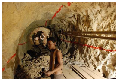
fig 7.3. Inside Mining tunnels
