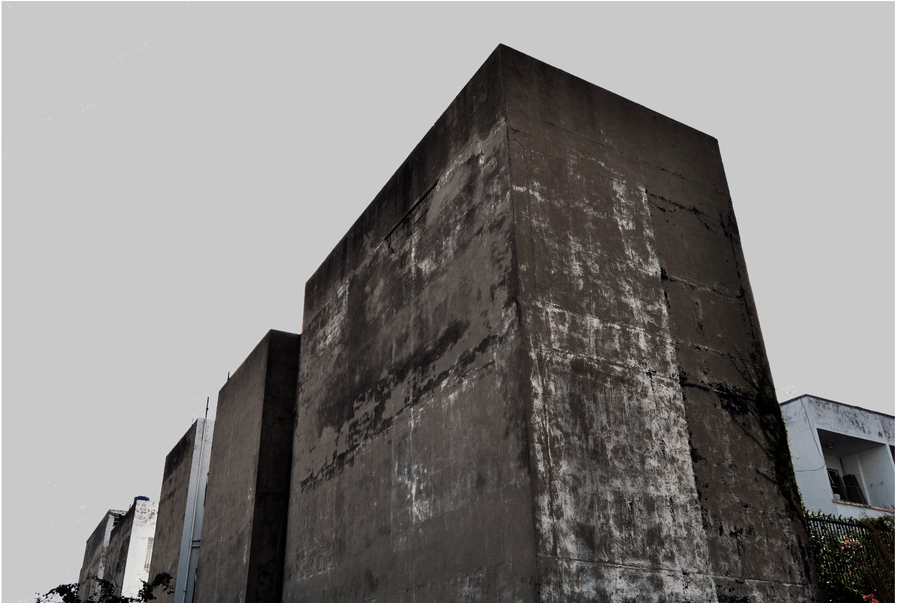
fig 4.25. Back of apartments bordering site along the North. (by Author, 2015)
