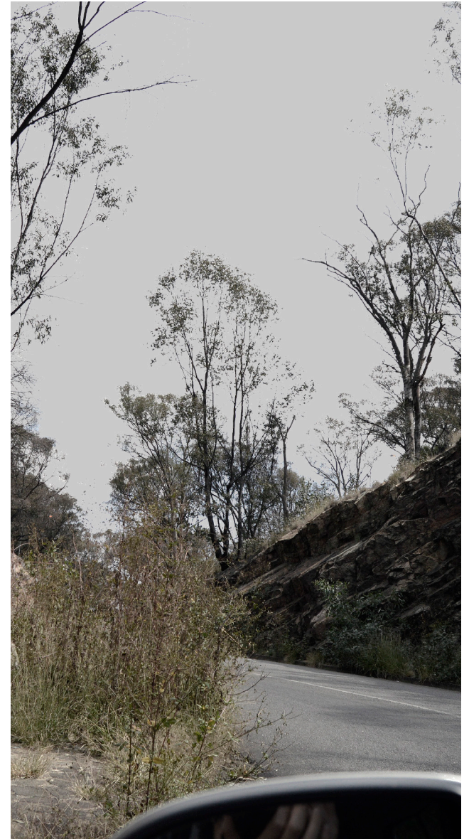
fig 4.17. View of exposed granite as a result of excavation. (by Author, 2015)
