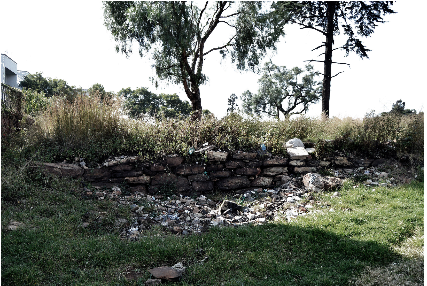
fig 4.11. Image of ruined dry packed stone wall on site. (by Author, 2015)
