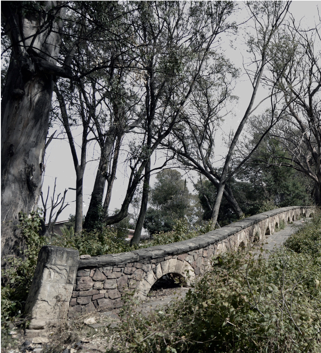
fig 4.16. Pedestrian walkway up winding road cut into ridge. (by Author, 2015)
