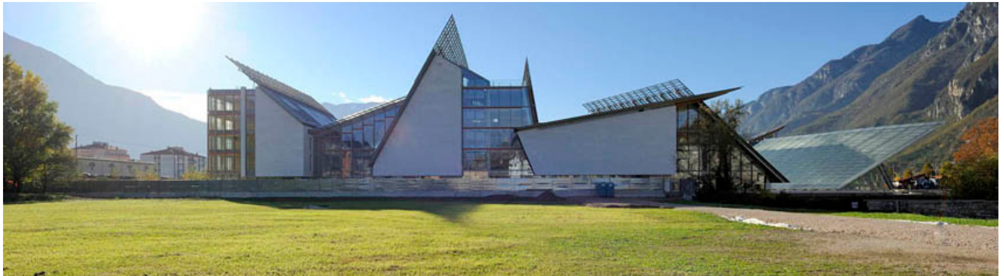
3.11_ Photo of the finished building ( http://www.archdaily.com/423101/muse-renzo-piano/522136ffe8e44e711f00001e-muse-renzo-piano-photo )
