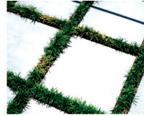
Grass between Concrete slabs
