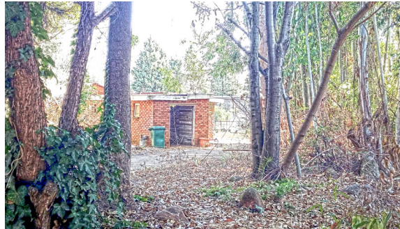
5.24_ Abandoned buildings in the zoo used for storage (Author, 2015).
