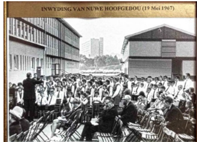
5.28_ Photos framed in the Prinshof school about the inauguration of the school, the new building being introduced (Author, 2015).
