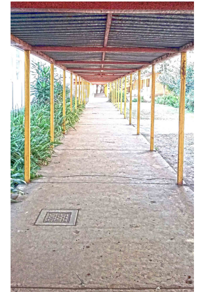
5.30_ The yellow columns is said to be visually stimulating for the visually impaired (Author, 2015).
