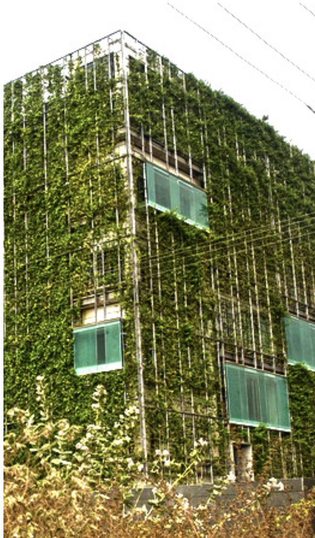
8.27_ Exterior view of the outer skin green facade ( http://rmaarchitects.com/architecture/kmc-corporate-office edited by author, 2015)
