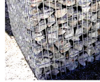
Gabion walls held together by welded wire mesh
