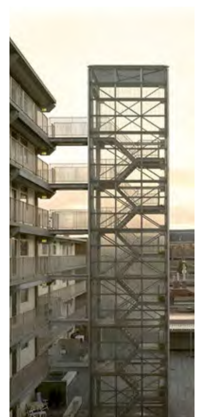
Figure 6.20: Steel staircase (Author 2015)
