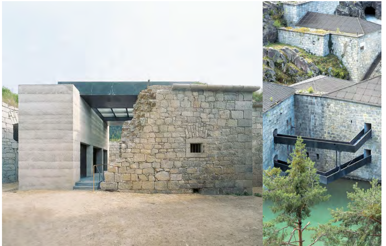
Figure 4.5: Façade interventions at the military fortress (Chemollo 2011)
