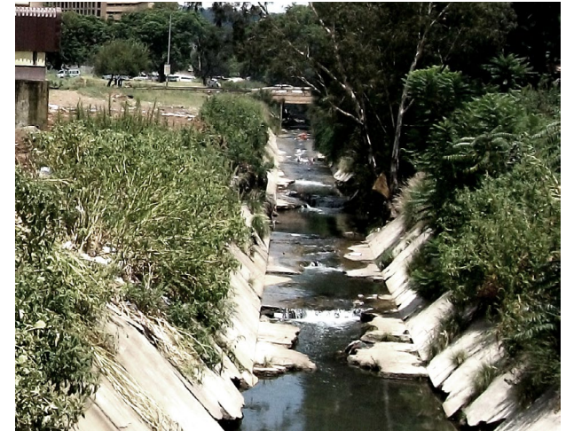
Figure 5.13. Steenhovenspruit goes underground (Author 2015)
