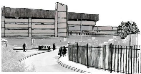
Figure 5.24. Belle Ombre Metro Station (Author 2015)
