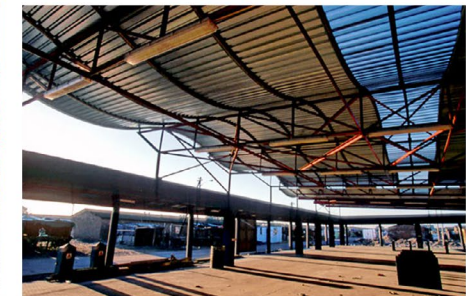
Figure 6.36. Central Meat market truss structure
