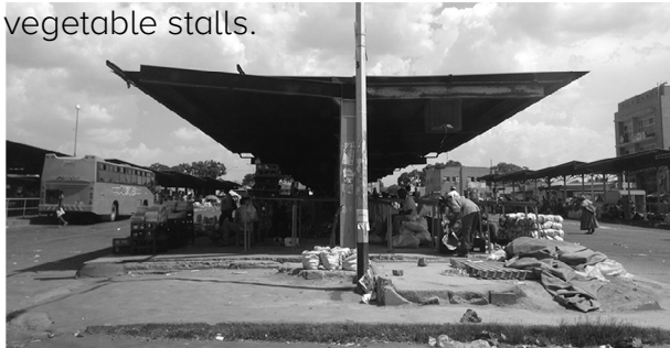
Figure 2.55. Reappropriated bus stop
