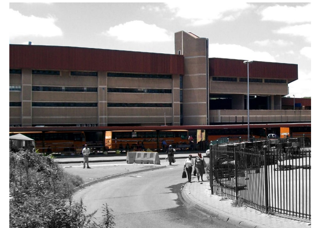
Figure 1.2. Belle Ombre Metro Station (Author 2015)
