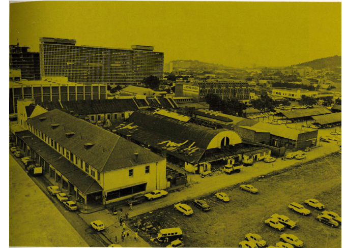
FIGURE 31 - LAST DAYS OF THE MARKET BUILDING (PRETORIANA)
