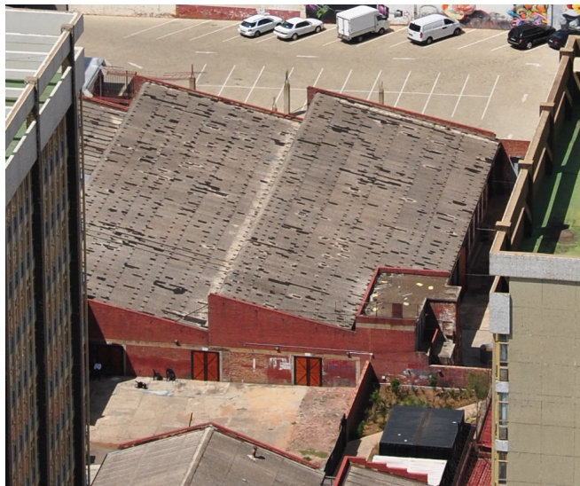
FIGURE 56 - ‘THE SHEDS’ HERITAGE BUILDING (AUTHOR, 2015)
