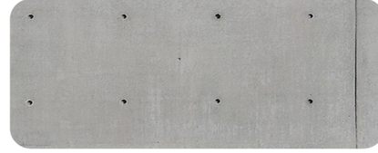
Off-shutter in-situ concrete walls and precast panels
