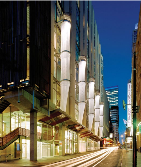
Figure 8.27: Photograph of the CH2 cooling towers lit up at night, Photo by Dianna Snape (CH2 2013)
