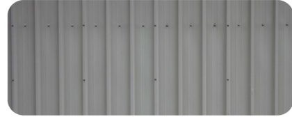
Concealed fix galvanised metal roof sheeting
