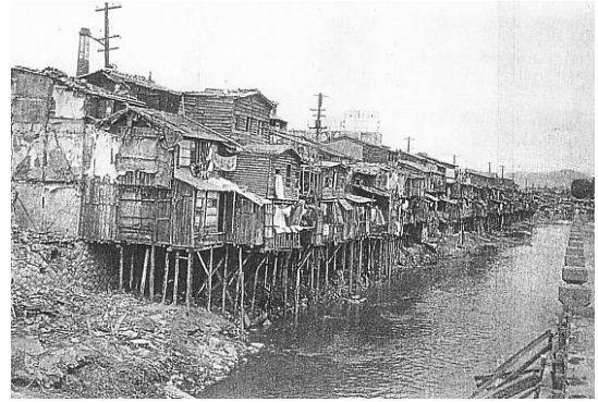
Figure 4.8: The Cheonggyecheon channel before the implementation restoration project, showing the implemented overpass in 1958.
