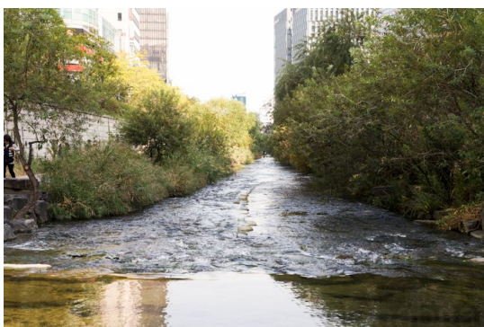
Figure 4.13: The termination of the constructed channel into a natural reserve.
