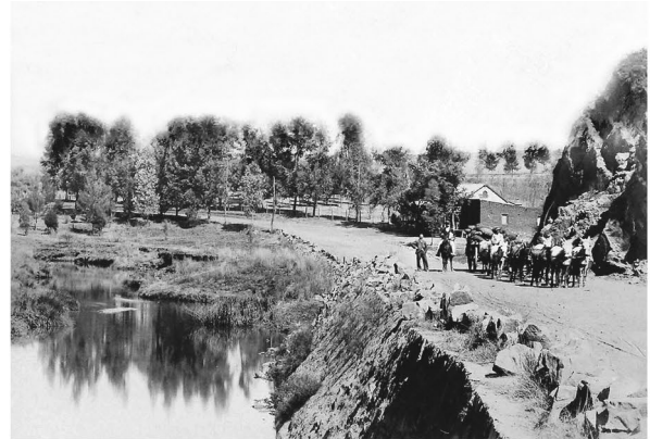
Figure 1.1 Crossing over the Apies River at Arcadia drift. (Hilton T)
