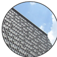
STEEL FRAME GLAZING
