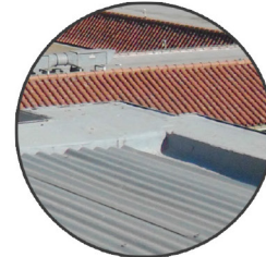
STEEL ROOF SHEETING
