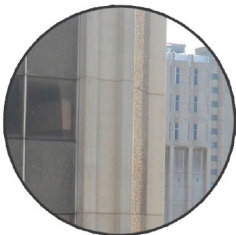
FLUTED CONCRETE COLUMNS
