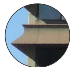
EXPOSED AGGREGATE CONCRETE CLADDING
