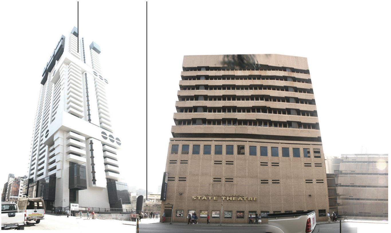
Figure 2.28 The northern edge of Pretorius Street. (Source: Author, 2015)
