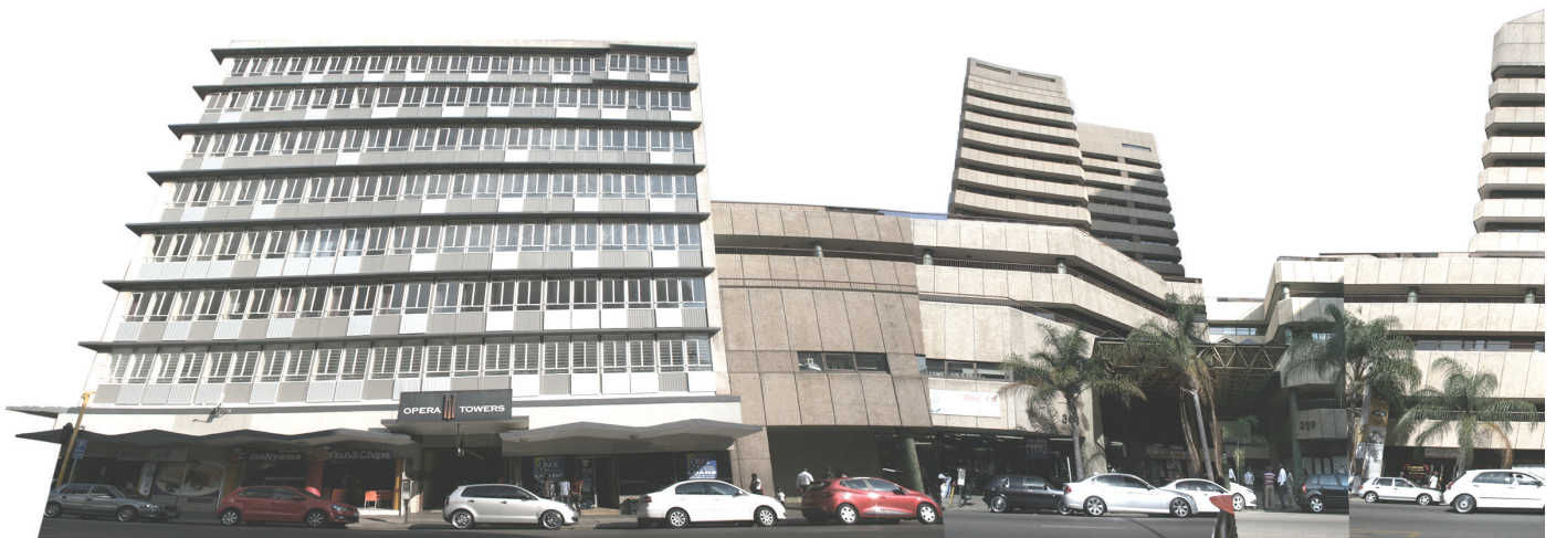
Figure 2.27 The southern edge of Pretorius Street. (Source: Author, 2015)
