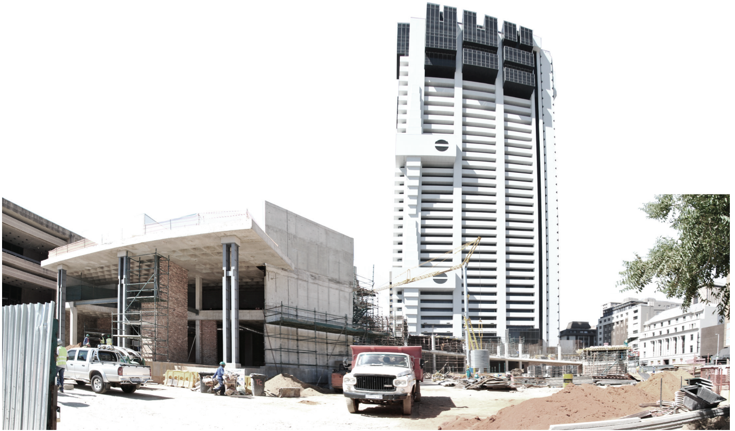
Figure 3.6 Construction of the Women's Living Memorial, March 2015. (Source: Author, 2015)
