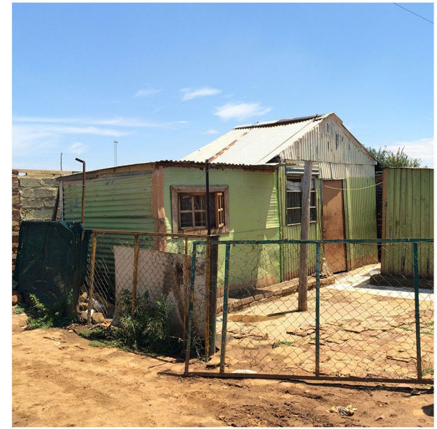
Fig. 2.6 The informal Settlement of Phumolong
