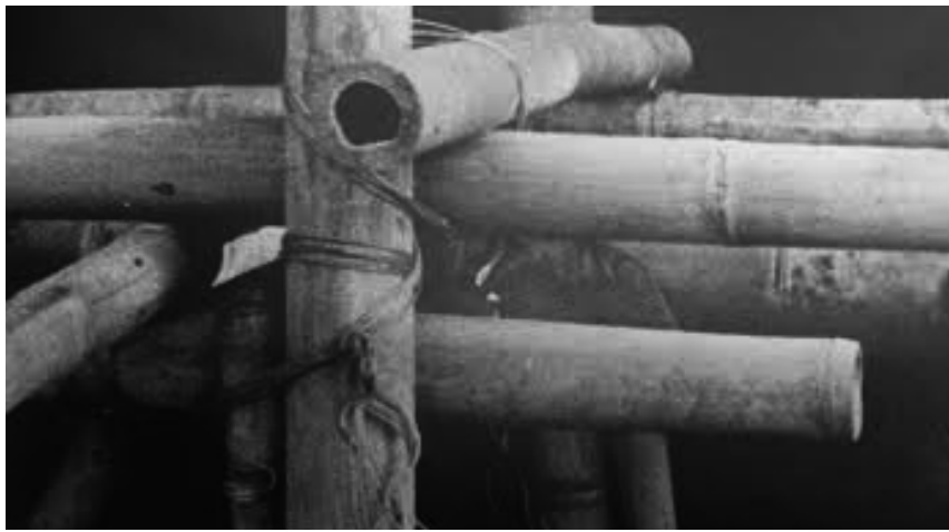
Figure 110 : Bamboo lashed joints, Photograph, Dunkleberg (1985) Figure 111 : Bamboo lashed joints, Photograph, Dunkleberg (1985) Figure 112 : Bamboo Scaffolding, Photograph, Dunkleberg (1985) Figure 113 : Bamboo lashed joints, Photograph, Dunkleberg (1985) Figure 114 : Bamboo lashed joints, Detail, Dunkleberg (1985) Figure 115 : Bamboo lashed joints, Detail, Dunkleberg (1985)
