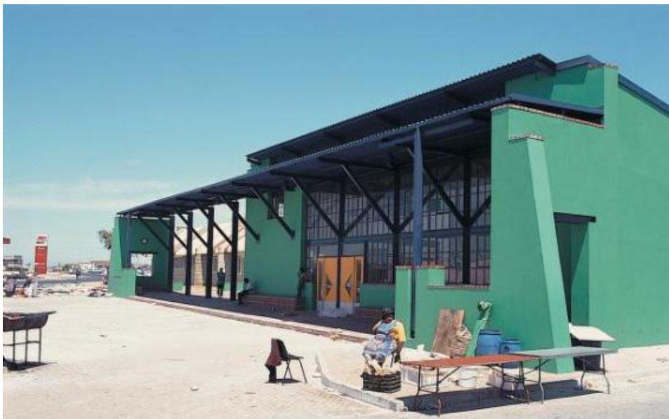
Figure 59 : Khayelitsha Service Centres And Pay Points, Photograph, Piet Louw Architects (2015) Providing for public interaction.
