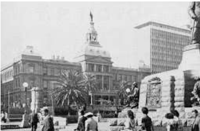
Figure 3.18 Photo of the Raadsaal (Council Chamber)
