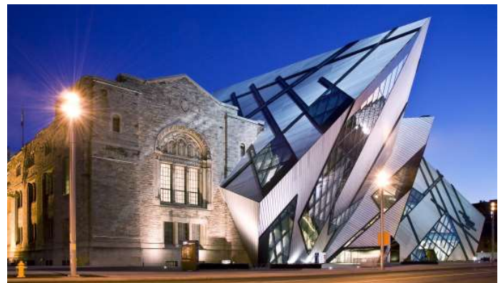
Figure 4.23 View of the building with the parasitic intervention
