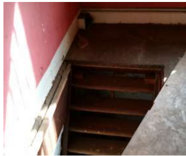
Figure 5.44 Existing trap-door to basement
