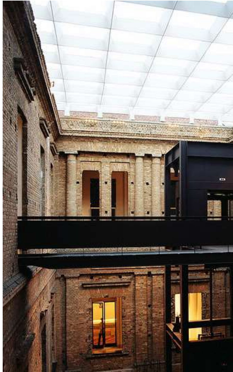
Figure 4.6 View of new walkways and how they connect the existing building fabric
