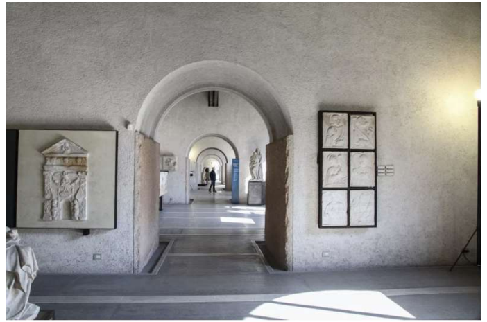
Figure 4.15 New floor meets existing walls
