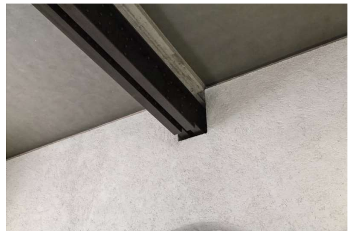
Figure 4.16 Beam connection with wall
