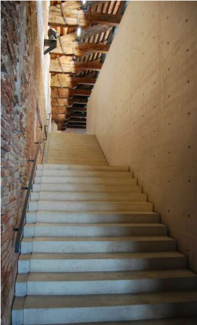
Figure 4.20 Concrete staircase intervention
