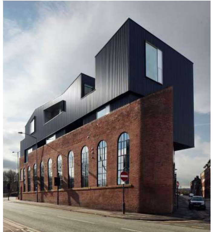
Figure 4.29 View of the building and the parasitic intervention
