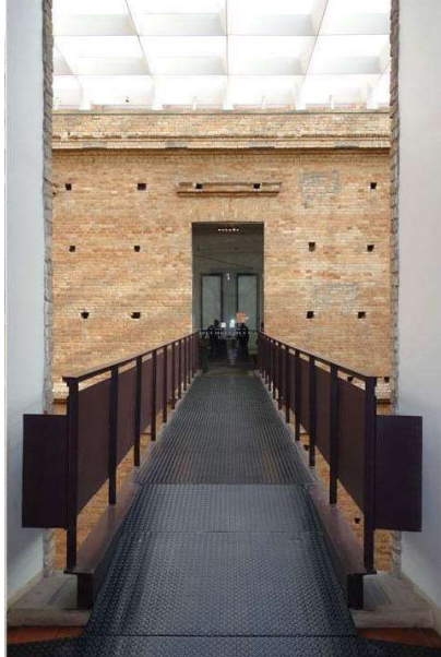
Figure 4.7 View of walkways
