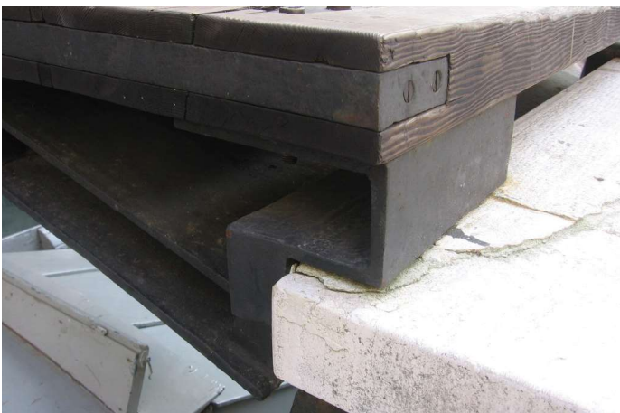
Figure 4.13 Detail of bridge connection
