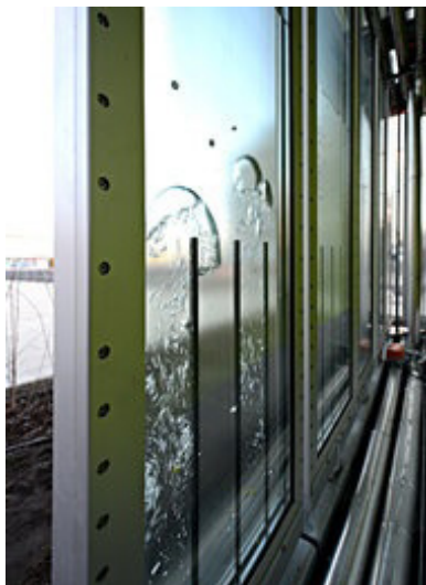
Figure 6.19 Algae bioreactor glass
