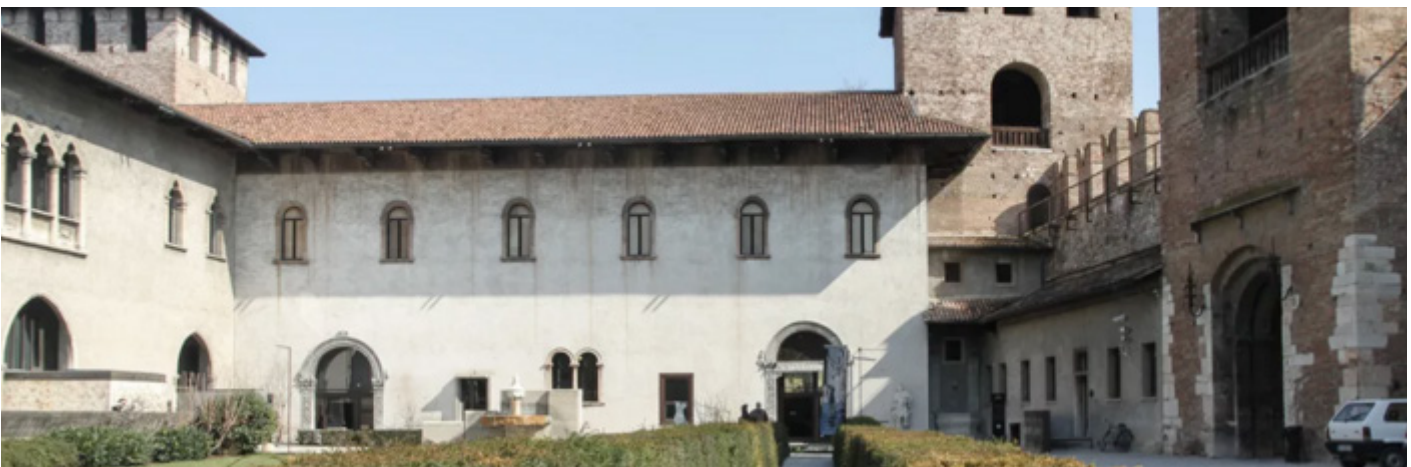
Figure 4.14 View of the building
