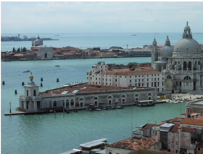
Figure 4.17 View of the building
