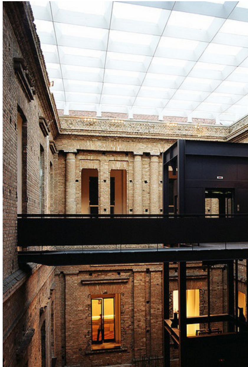
Figure 4.6 View of new walkways and how they connect the existing building fabric
