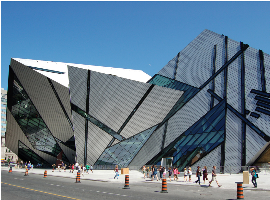
Figure 4.24 View of the exterior parasitic intervention
