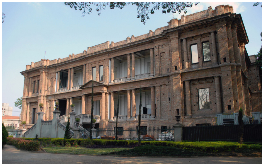
Figure 4.9 View of the building
