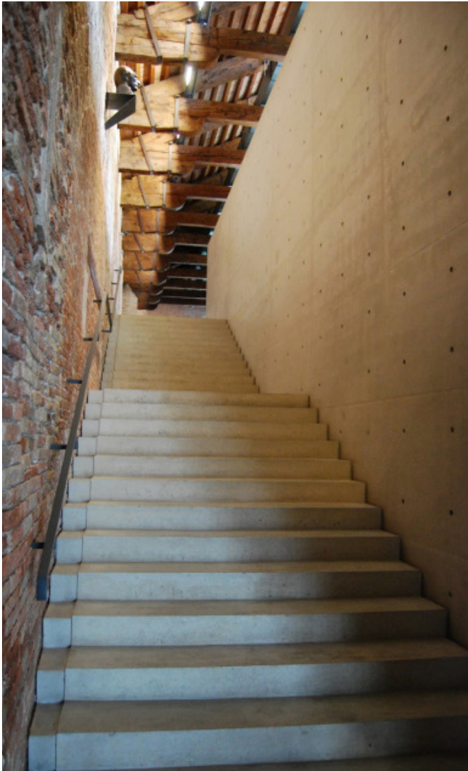
Figure 4.20 Concrete staircase intervention
