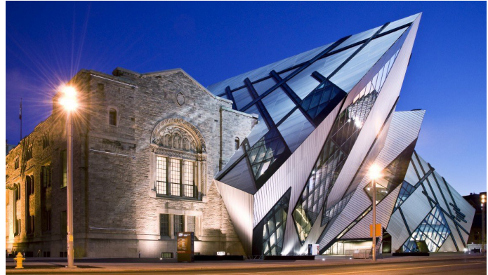
Figure 4.23 View of the building with the parasitic intervention
