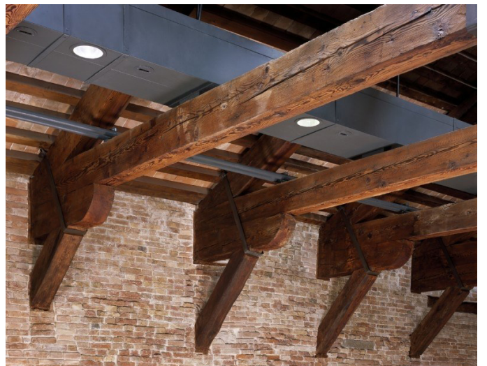
Figure 4.21 Beam connection to the wall
