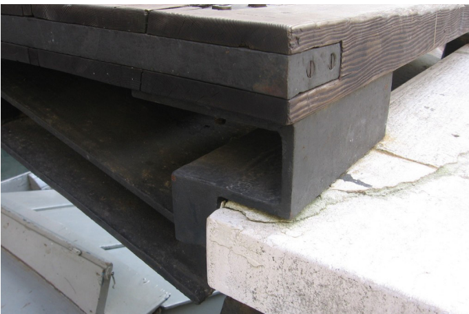
Figure 4.13 Detail of bridge connection
