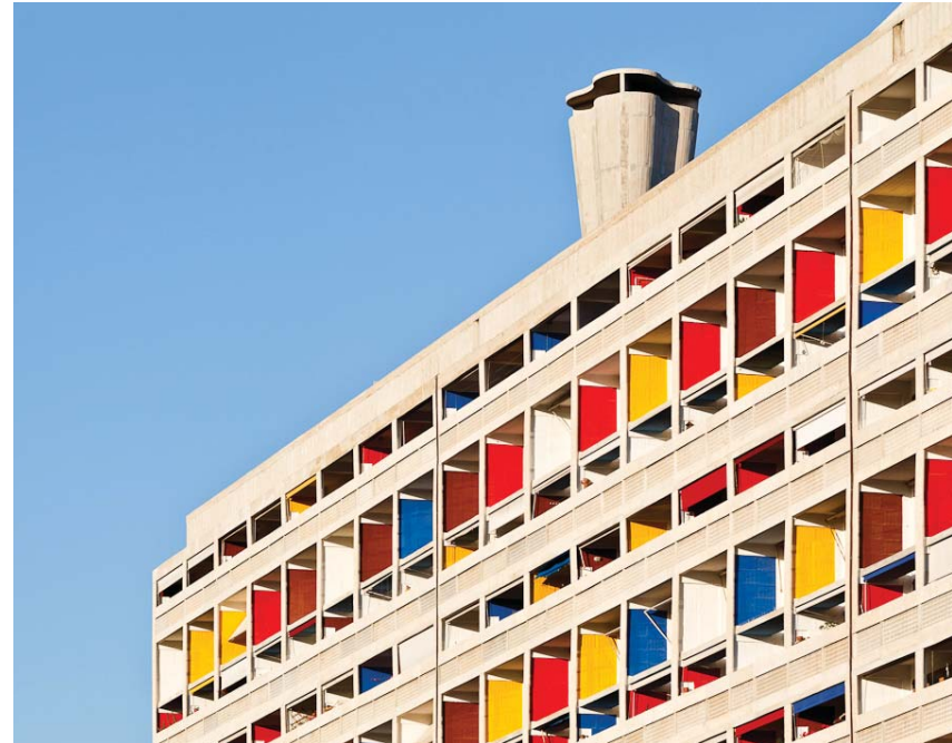
Figure 4.1 Exterior facade of the Unite d' Habitation (Uncube magazine 2013).
