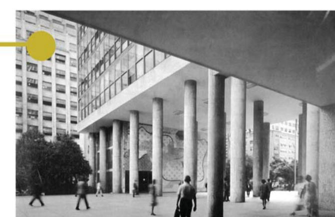
Figure 2.34 Ministry of Education building, Rio de Janeiro (Studyblue, [S.a.]).
