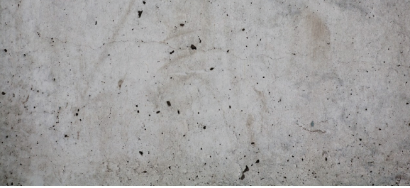
Portland cement concrete
