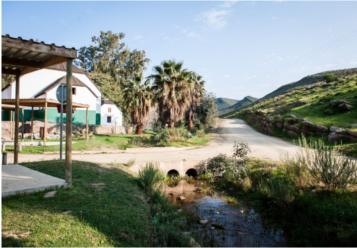
Fig. 7.46 Service bridge (Franklin 2015)
