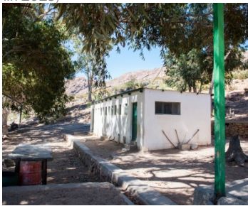
Fig. 6.32 New toilets on school yard (Franklin 2015)
