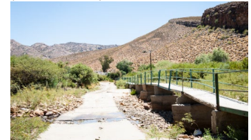
Fig. 2.35 Wupperthal, pedestrian bridge (Franklin 2015)
