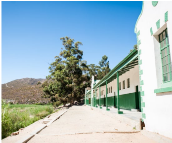
Fig. 6.30 School building (Franklin 2015)
