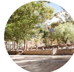
2. Retaining rock walls
