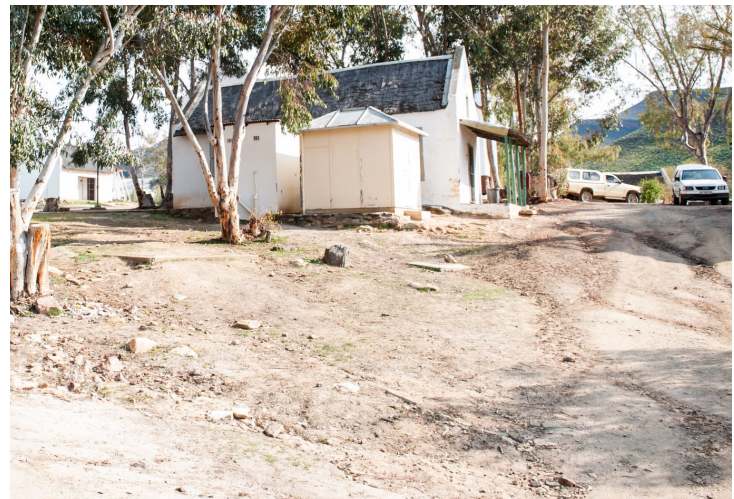
Fig. 7.49 Erosion next to post office (Franklin 2015)
