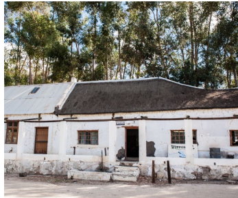
Fig. 6.33 Shoe factory building (Franklin 2015)
